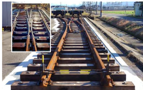
Fig. 1. Experimental track with turnout.
