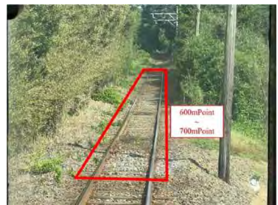
Fig.11. Section where line maintenance work
