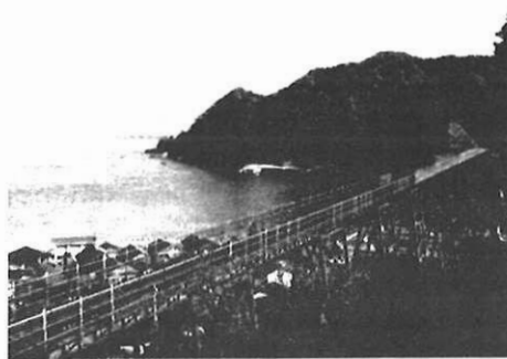
Fig.1 Appearance of the target bridge
