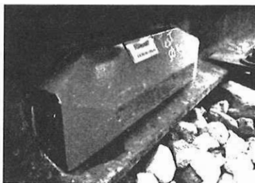
Fig.1 Installation of RSM.
