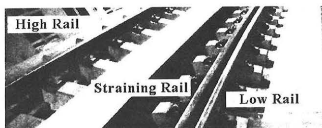
Fig.1 Track Structure of Imazatosuji Line
