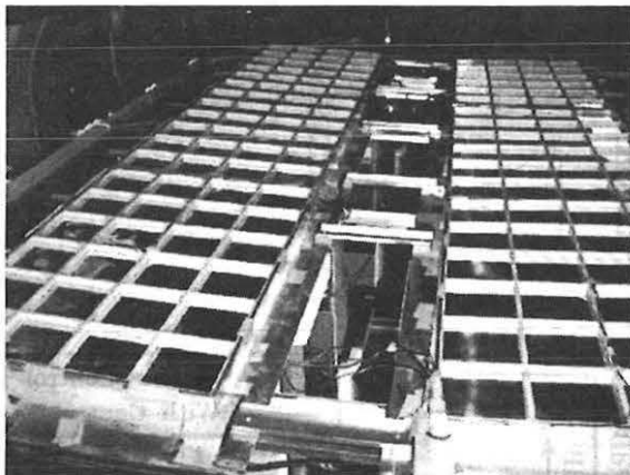
Fig.7 Installed condition of the noise control panels on the back of interior ceil panel
