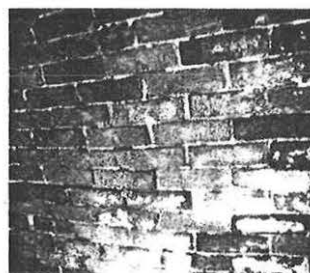
Fig.6 harmful alteration of brick
