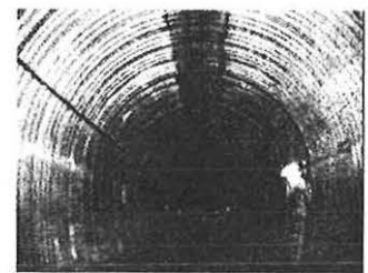
Fig.14 example of reinforcement work
