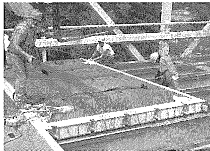
Photo 1 Bridge Decks of Sandwich Panels made by Pultrusion and Injection Core (by Eric Munley)
