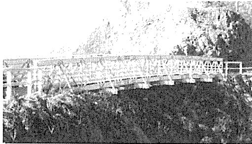
Fig. 1 24 m long FRP pedestrian truss bridge
