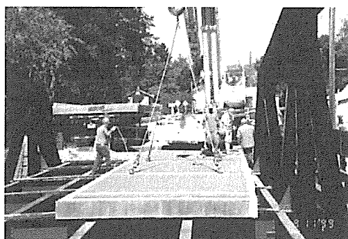
Fig. 15 Installation of molded panels on steel stringer bridge (photo: J. O'Connor)
