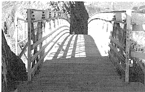
Fig. 2 End view of pultruded truss bridge
