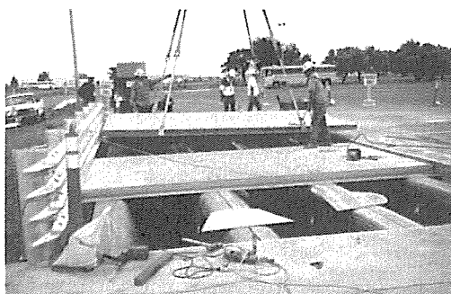
Fig. 14. First FRP deck panel installed in the USA in 1995 (photo: Martin Marietta Composites)
