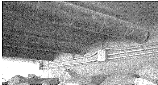
Fig. 20 Hybrid FRP tube/concrete girders in California
