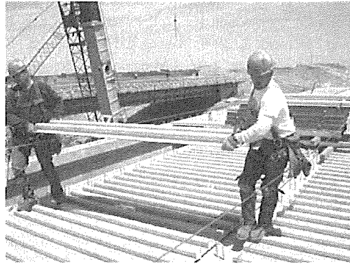
Fig. 21 FRP SIP/reinforcement panel being placed.
