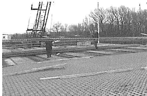
Fig. 22 Installation of very large pultruded grids
