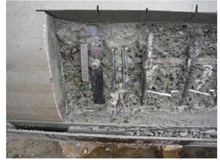
(c) 支圧板背面・補強鉄筋周囲
