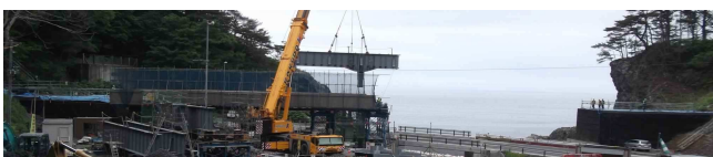
(c)起点方径間鋼桁架設
