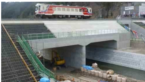
(a)松前川橋梁
