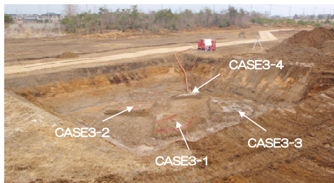
図-13 掘起し改良体全景
