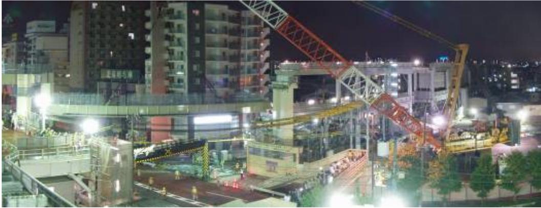
写真-7 GA2桁(2F)架設状況(750tCC)
