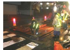
1) Construction condition of Japan (Night time)
