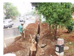
2) Construction condition of Indonesia (Day time)
