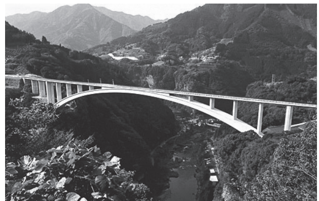
Fig.5 “Tensho Ohashi”, existing bridge
