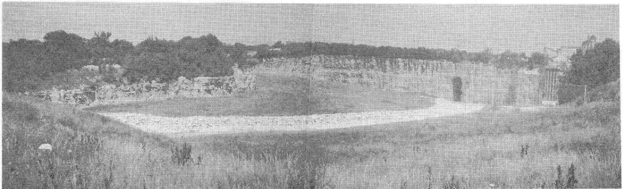
Photo 1 Elmhurst Quarry Flood Control Facility.
