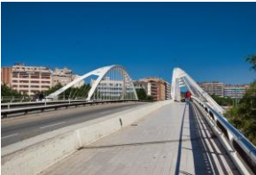
図-31 narrow (Bac de Roda Bridge)
