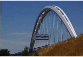
図-32 tear (A-12 Ebro River Bridge)
