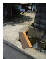
④ 2015, Kita, Kizugawa, additional, bridge
