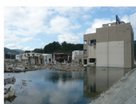
② **, 2011, Kita, Sanriku, disastrous, water
