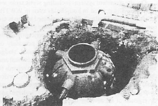
Photo 7 On-site treatment system for both black and gray water being installed in Chiang Mai University campus
