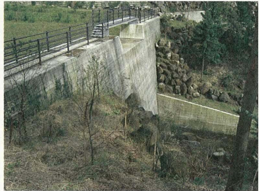
Photo 4 Rocks layered on the side of the concrete dam
