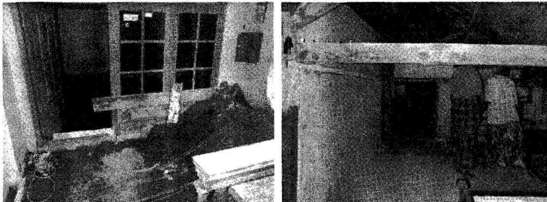
Photo 5, 6 Adaptation, by heightening the ground floor by sand, Semarang
