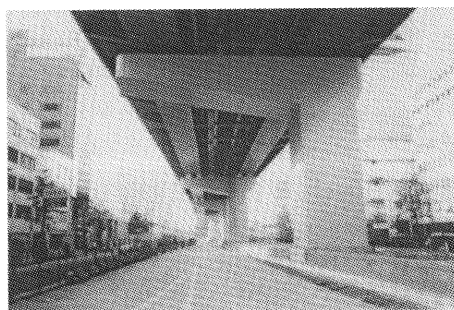
Fig.1 Inverted L-shaped steel bridge pier (Nagoya Expressway)
