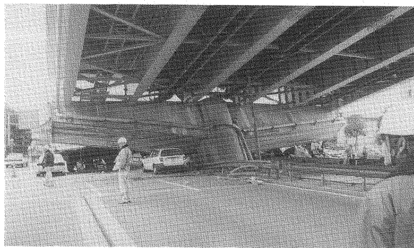
Photo 3 Failure of Reinforced Concrete Pier, Takashio
