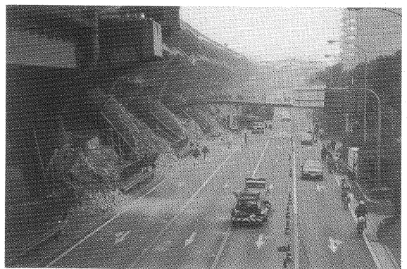
Photo 1 Collapse of 18-span Bridges from Kobe Side, Fukae, Route 3, Kobe Line, Hanshin Expressway
