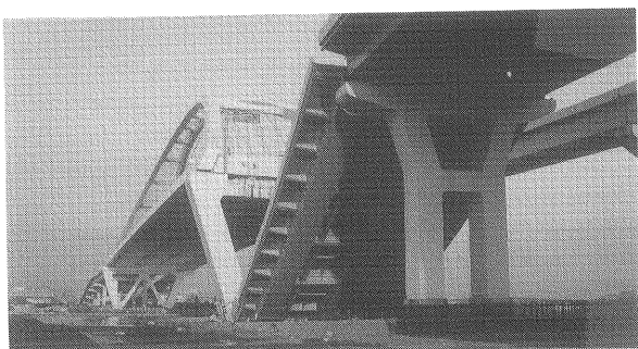
Photo 5 Collapse of an Approaching Bridge to Nishinomiya Bridge, Route 5, Bay Shore Line, Hanshin Expressway
