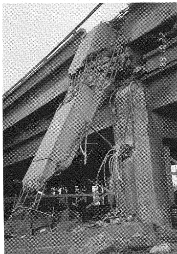
Photo.2 Collapse of the Cypress Double-Deck Bridge on the opposite side of Photo.1
