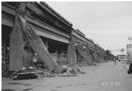
Photo.1 Collapse of the Cypress Double-Deck Bridge on Interstate 880-Line
