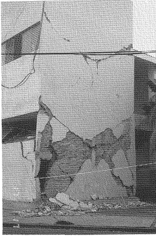
Photo 3 Typical Shear Cracks in a Brick Wall (Mexico Earthquake 1985).
