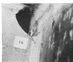
Fig. 19 Fatigue crack at the scallop of the vertical stiffener.
