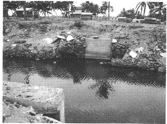
Photo 10 Supporting base columns of a damaged bridge
