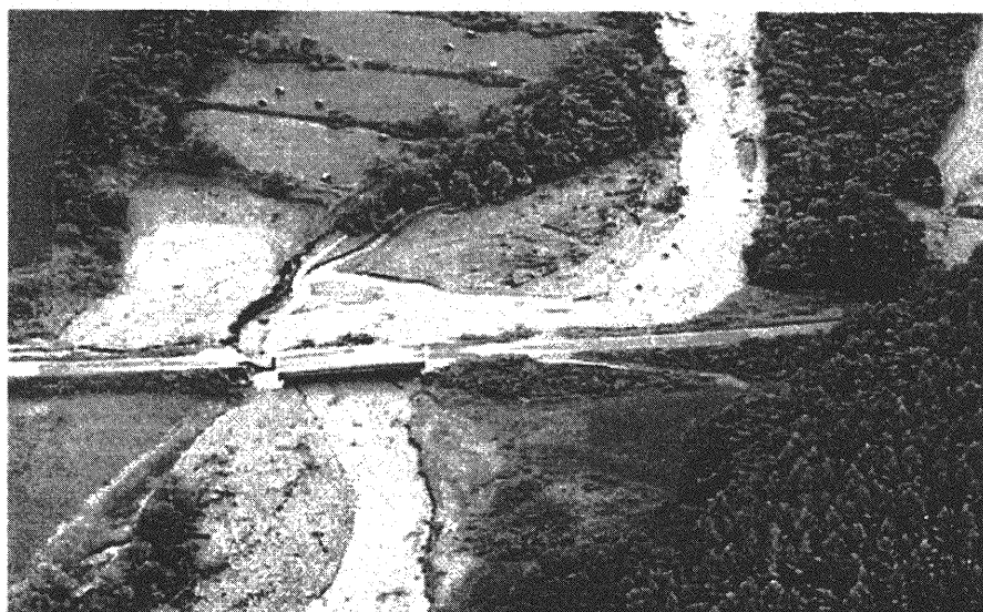
Fig. 11 Damage to the Eishin Bridge due to the flood (Photograph offer: Shin Engineering Consultants Company, Limited Company)
