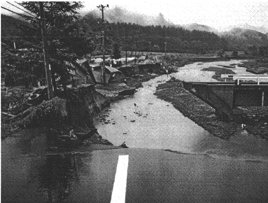
Fig. 4 Collapsed road due to progression of bank erosion to the backfill material of the abutment (Photograph offer: Hokkaido Prefecture Government Office)
