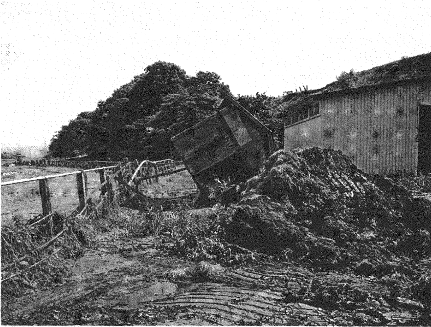
Fig. 3 Collapsed barn on the lower stream of the Appetsu River due to the flood
