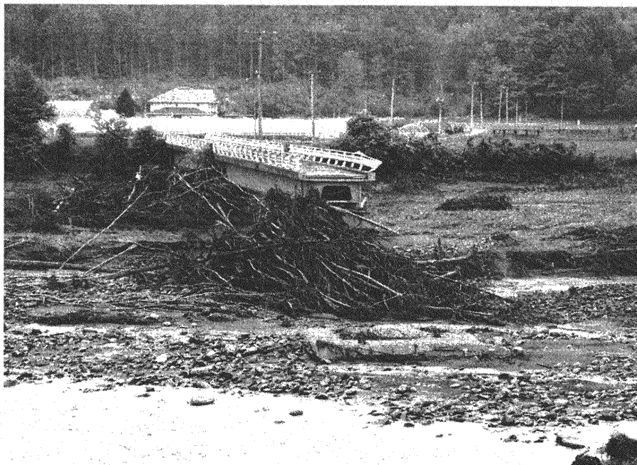
Fig. 10 Abushitoenai Bridge of 4-span continuous bridge washed away due to driftwood caught in the bridge pier and bridge girder
