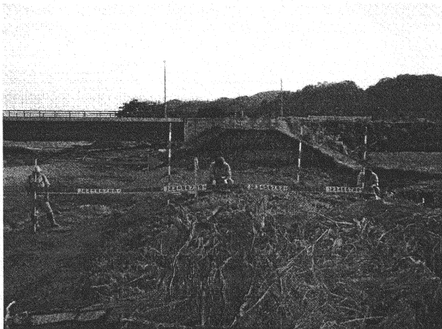
Fig. 7 Flood levee failure in the upstream side of the Higashikawaoohashi Bridge (Photograph offer: Hokkaido Prefecture Government Office)
