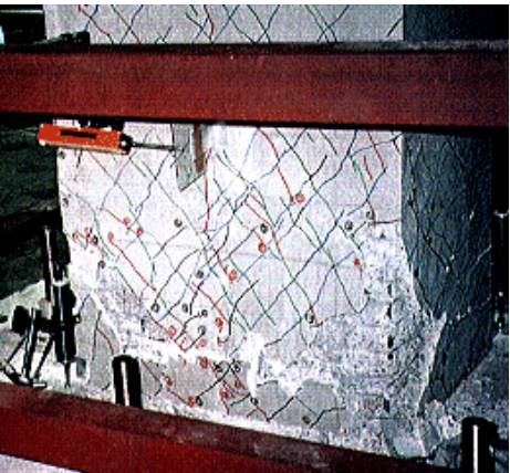
Photo 3 Specimen 2 Damage at Base
