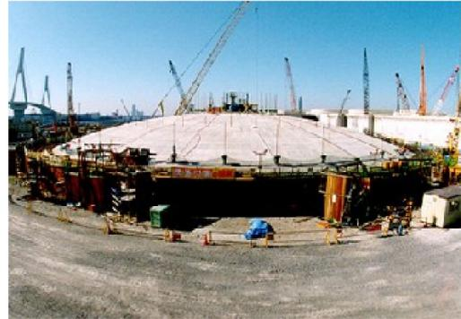
**Photo 4** Concrete Dome Roof during Curing
