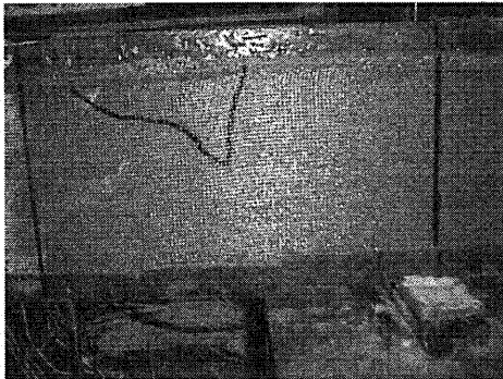
(a) Photograph of Shear Failure in 97-S-A
