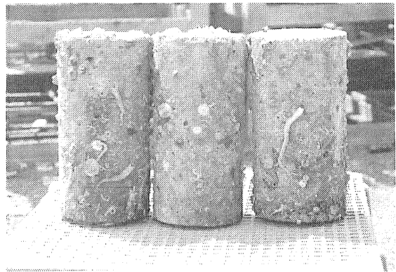
Photo. 1 Appearance of Cylinder Specimens at 10 Years of Exposure (Splash Zone)
