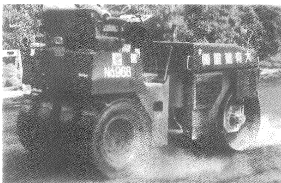
Photo 3 Roller Compaction for Asphalt Concrete
