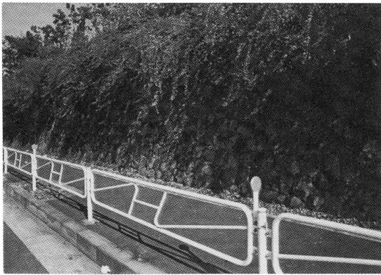
(iii) Retaining wall using blocks finished like natural stone, with trees planted at close intervals on the top of the slope
