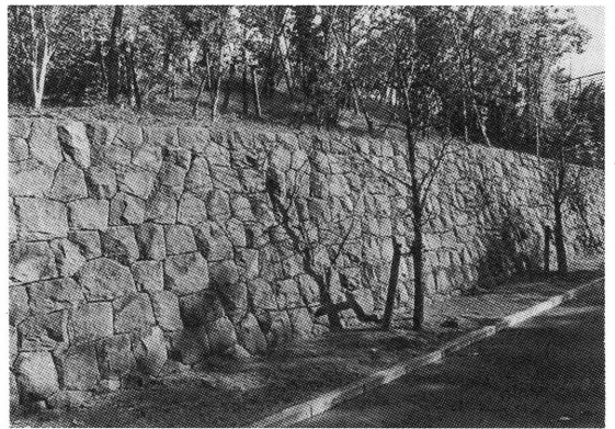
(iv) Retaining wall using blocks finished like natural stone, with trees planted on the top of the slope
