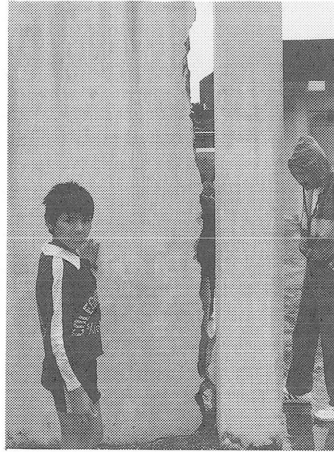
Photo 4 No Connecting Steel Bar between the Column and Wall (Ecuador Earthquake 1987).
