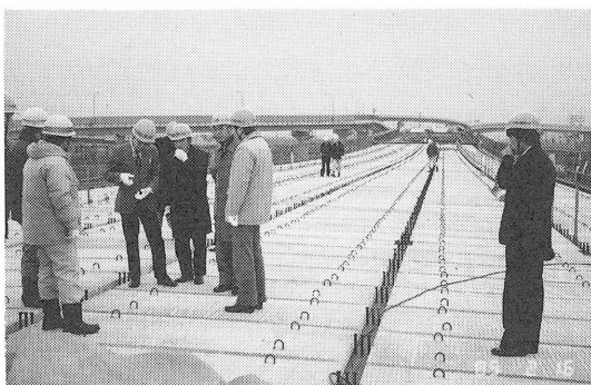
Photo. 3 Application of PCC Panel to Steel Composite Bridge
