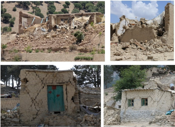
Fig.5 Views of the failed simple adobe buildings.
