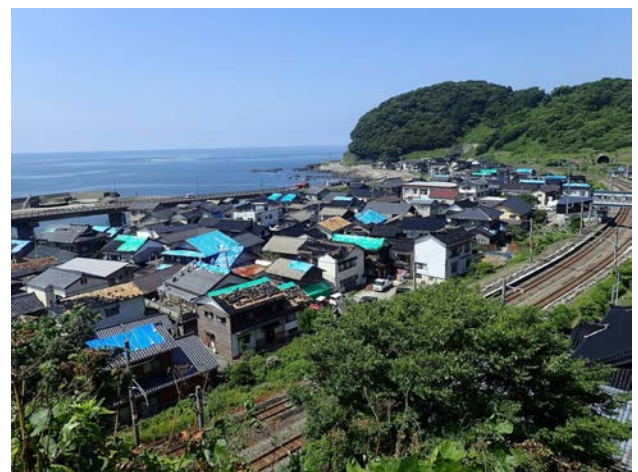
Fig.5 Damage situation of roof tile in Koiwagawa on June 20 th . Some houses have begun to have repaired.
