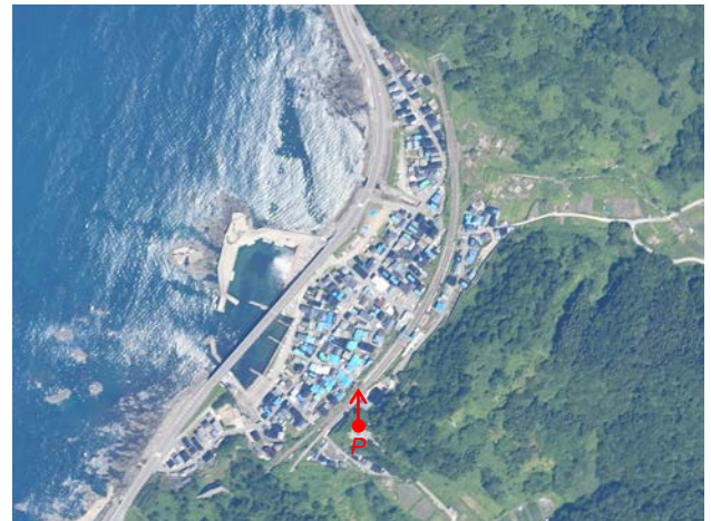
Fig.4 Aerial photograph in Koiwagawa on June 26 th , 2019 8) . There are many houses covered with blue sheet. In this study, houses covered with blue sheets were considered as damaged houses.
