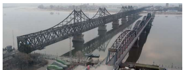
Fig.2 Present Yalu river bridge 1)
