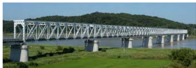
Fig.1 Present Imjin river bridge 1)
