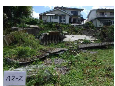
(i)L型擁壁の倒壊 (南阿蘇村)
