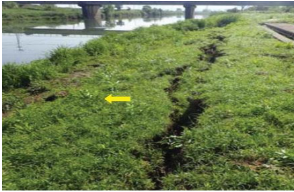
Fig.1 Lateral Spreading during 2016 Kumamoto Earthquake.
