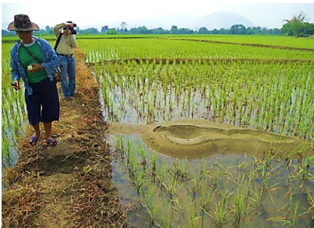
Fig.1-b Liquefaction evidences on paddy field due to Tarlay Earthquake (Tapanalungkorn and Teachavorasinskun. 3) )
