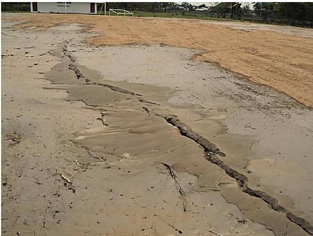
Fig.1-a Liquefaction evidences on free field due to Tarlay Earthquake (Ruangrassamee et al. 1) )
