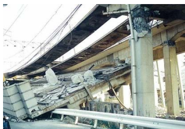
(a) 損傷度Aの被害
