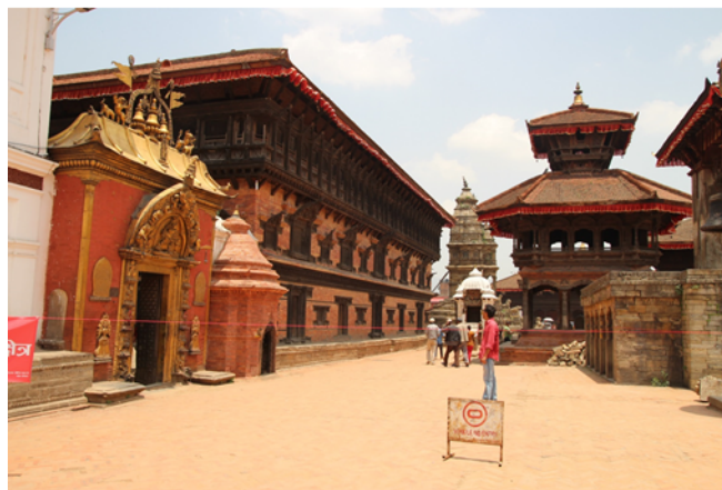
After the earthquake
