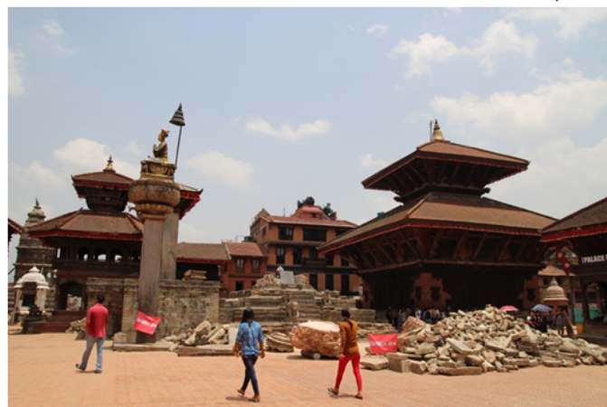
After the earthquake
