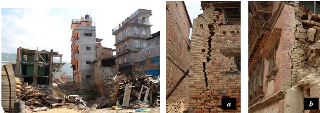
Fig.3.10 The damage to RC structures was generally minor. These structures were mainly five to six story buildings. Many of the non-engineered masonry structures that experienced complete collapse or partial damage were two to four story buildings in Sankhu ( left ). Damage in non-engineered masonry structures was initiated by vertical cracks in the corners of the buildings ( a ), which contained no RC columns ( b ). (Photo. by T. Ohsumi).
