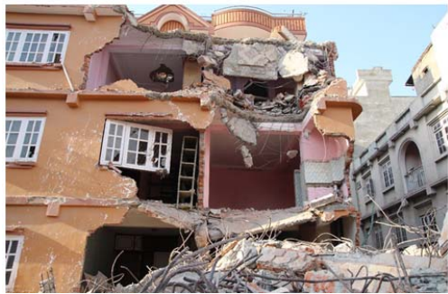
Fig.3.18 At the branch point of the Bagmati River and the Transformer River, collapsed building fell onto and destroyed the next building (Photo. by T. Ohsumi). OpenStreetMap https://www.openstreetmap.org/
