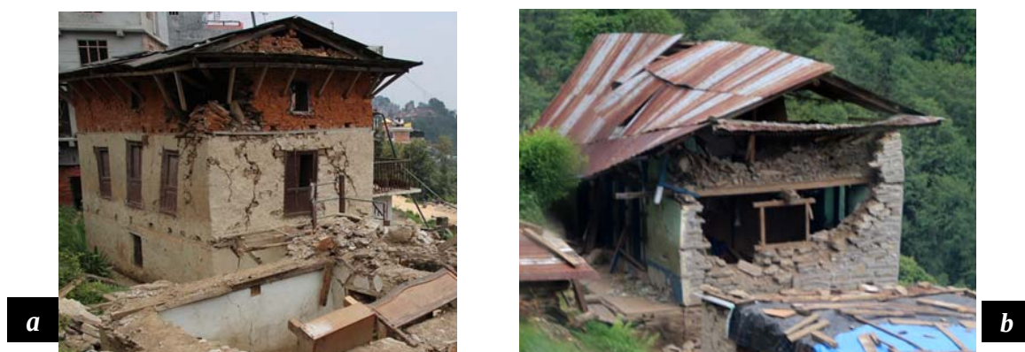
Fig.5.1 Adobe style houses (a) and Stone style house (b) in Charikot, (Photo. by T. Ohsumi)
