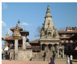
Fig.3.2 Reinforced Chayslin Duga temple (a and b: left) by steel frame, Vatsala temple (b:center and c) was destroyed and Yaksheshvara temple (b:right) survived, before / after 2015 earthquake in Bhaktapur (Photo. by T. Ohsumi).
