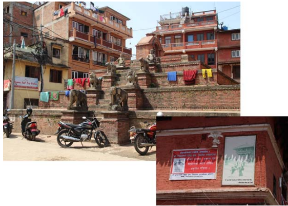
Fig.3.3 This temple in Bhaktapur collapsed in 1934 earthquake, but has not been rebuilt (Photo. by T. Ohsu-mi).
