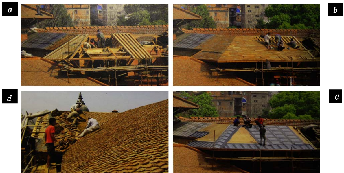
Fig3.4 Renovation of the structure and the cover of the roof was carried out in 2011.
