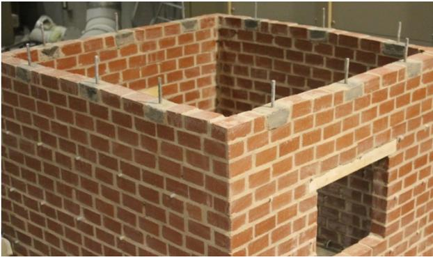
Fig 2. Connecting bricks for roof truss at the top most layer
