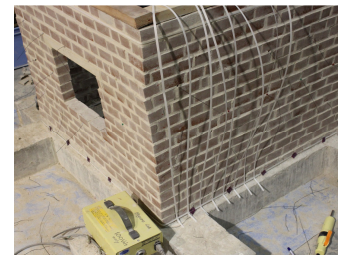
Fig.4 Attachment of Vertical PP-band with horizontal
