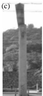
**Fig.4** Earthquake damage to the first gate of Sumoto Hachiman Shrine; (a) Front view of gate; (b) Focused damaged portion; (c) Side view of gate showing sliding of horizontal member.
