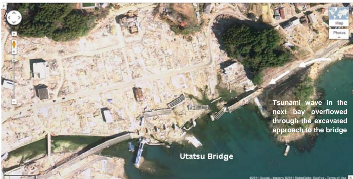
Figure 14 Decks of Utatsu Bridge carried inland (Satellite imagery from Google Map)
