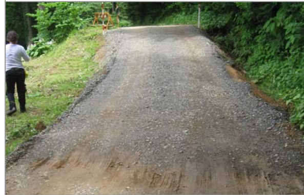
Figure 13. Fault dislocations along Idosawa Fault. The road meandering around the mountain was bisected at a number of locations ( 36^{\circ}59'41.5'' , 140^{\circ}41'12.8'' (upper photo) 36^{\circ}58'44.4'' , 140^{\circ}41'42.4'' (lower photo)).
