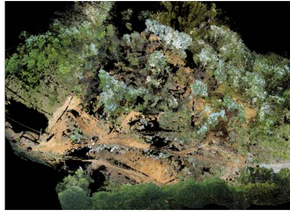
Figure 4. Landform of the lower half of the landslide mass obtained by ground LiDAR survey
