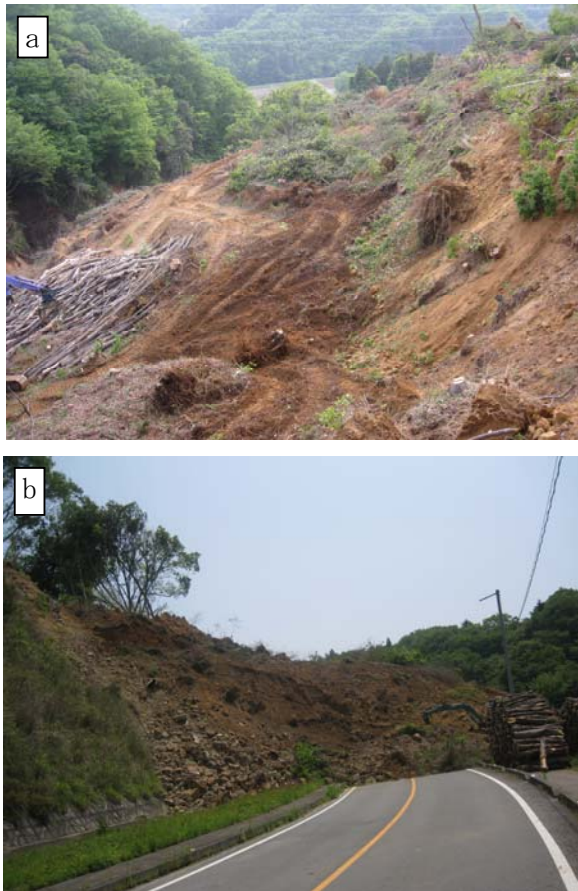
Figure 3. A view of the landslide from a) right and b) left ( 37^{\circ}00'00.3'' , 140^{\circ}47'14.5'' ).
