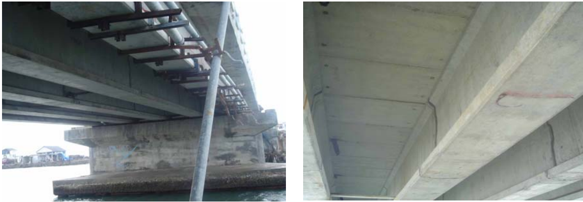
Figure 3. Prestressed-concrete girders supporting a deck
