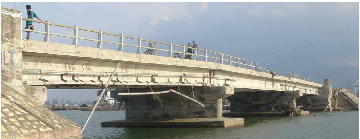
Figure 2. Three-span Ulee Lheue Bridge (No.2), March 03, 2005
