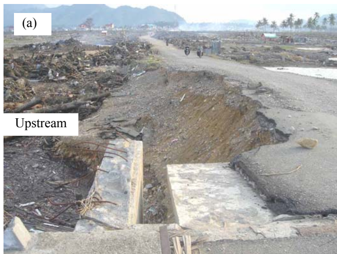
Figure 8. Scouring at the upstream side (a) North abutment and (b) South abutment
